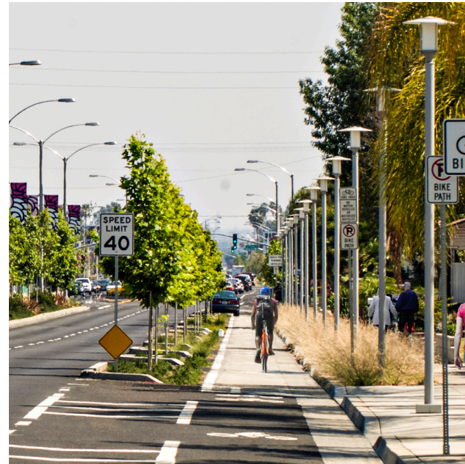
Protected Bike Lane on Rosemead Blvd. -Temple City, CA Source: Gruen Associates
