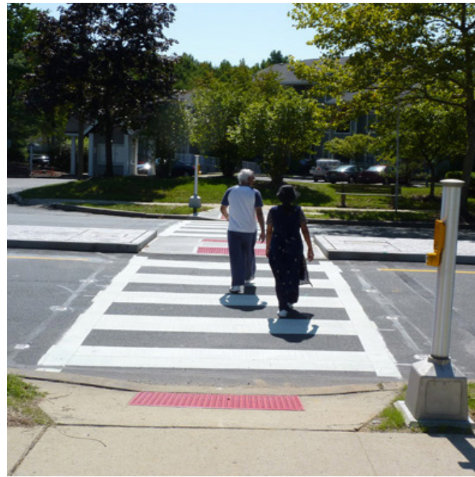
Pedestrian Refuge Island at mid-block crossing Source: Gruen Associates
