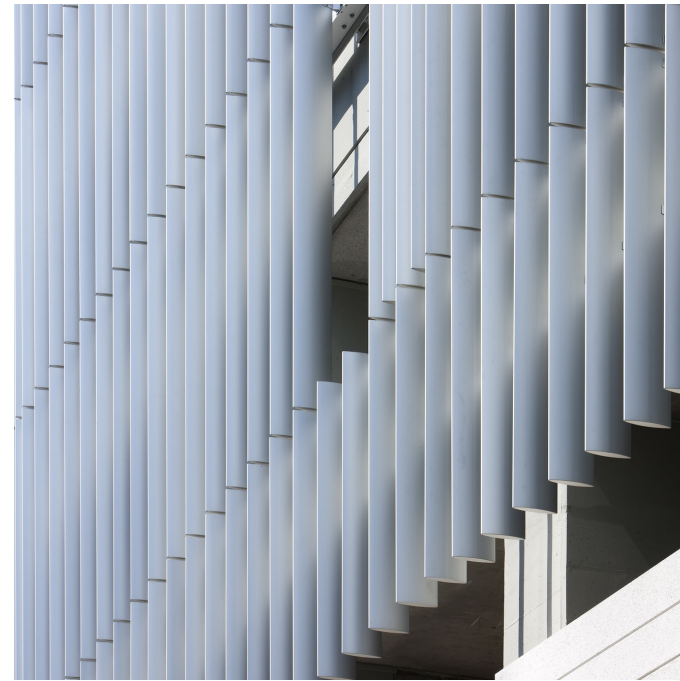
Green Square Parking Deck - Pearce Brinkley Cease + Lee Raleigh, North Carolina Source: http://www.clarknexsen.com/
