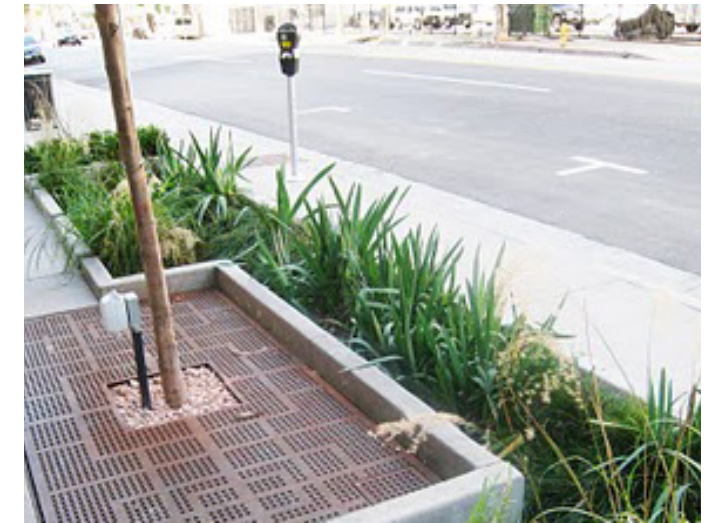
Bioswale parkways in Public Right of Way, Downtown L.A. Source: Gruen Associates
