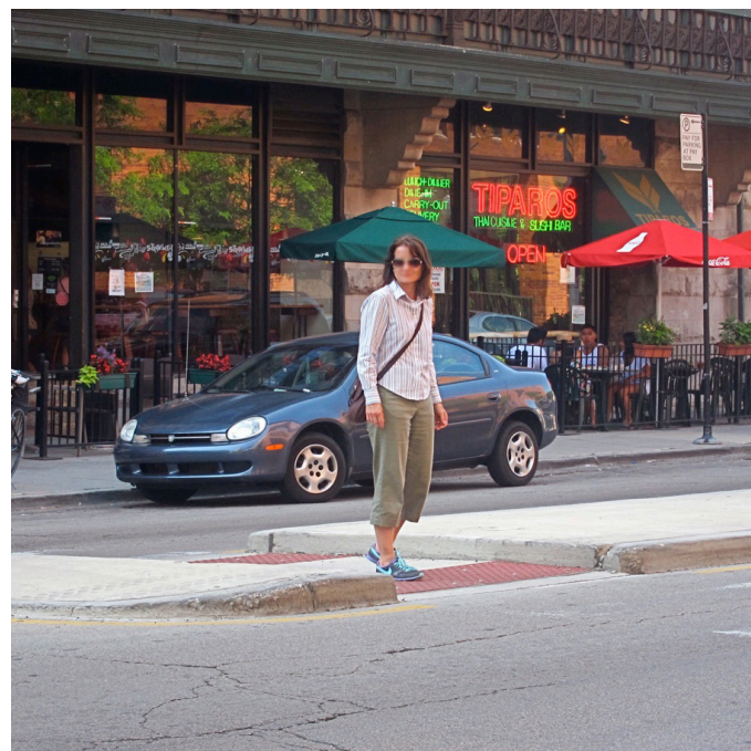
Pedestrian island on Clark Street, Chicago, Illinois Source: Bike Walk Lincoln Park
