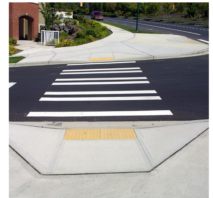
Wausau pavers, ADA-70 truncated dome pattern Source: http://www.pedbikesafe.org
