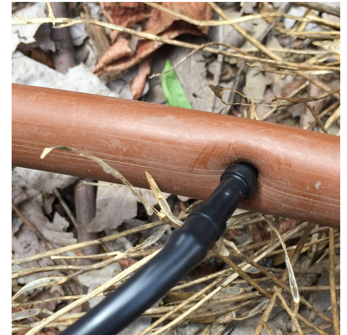
Drip irrigation system Source: Gruen Associates
