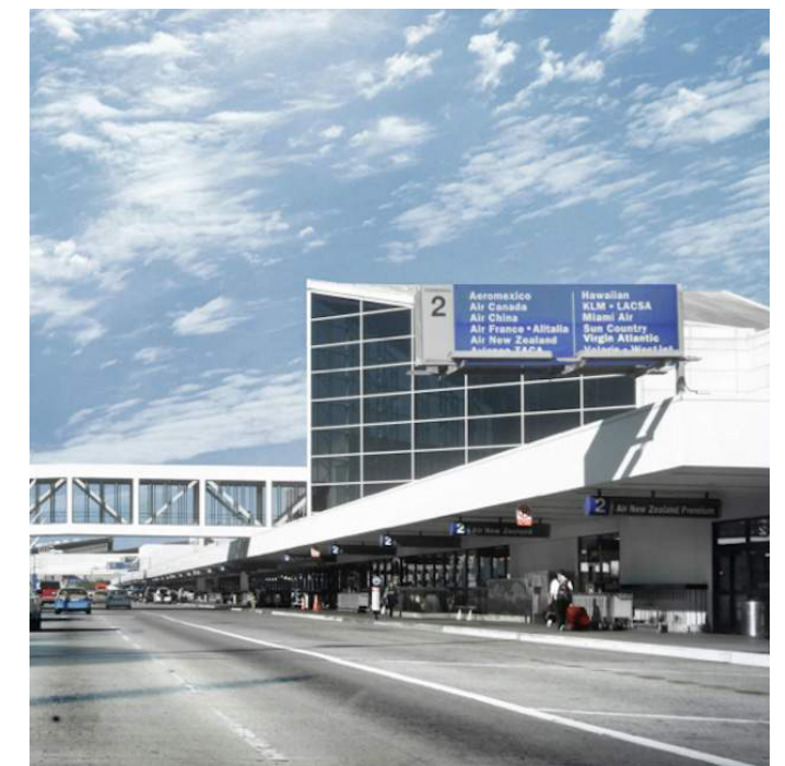
LAX CTA and Airport-Related Facilities: View of Terminal 2 in the LAX CTA.
