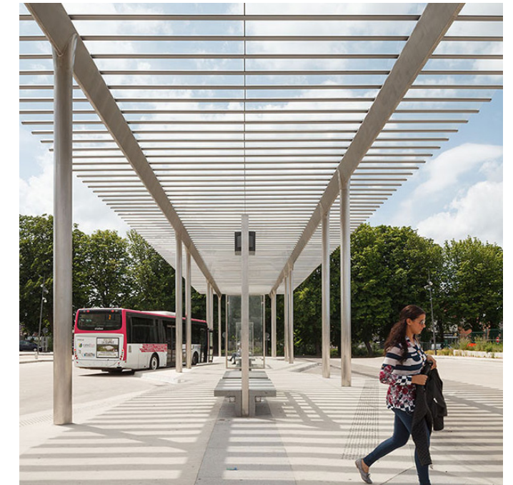
St Omer Station Canopy - Ney Partners, St Omer, France Source: http://www.ney.be/
