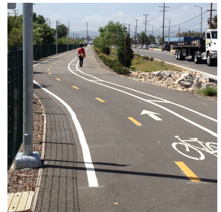
Metro Orange Line multi-use path along Canoga Blvd Source: Gruen Associates
