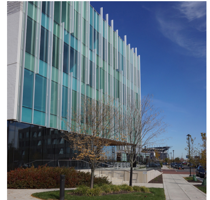
A glass curtain with metal fins create an iconic glass box entryway adjacent to the sidewalk.
