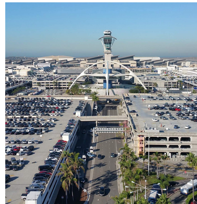
LAX CTA and Airport-Related Facilities: View looking west of the LAX CTA.
