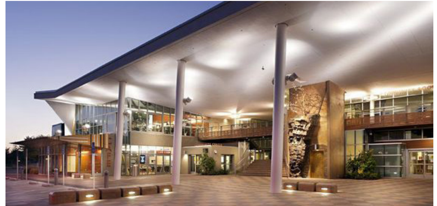
Bascom Library and Community Center - Rob Quigley -San Jose, CA Source: http://robquigley.com
